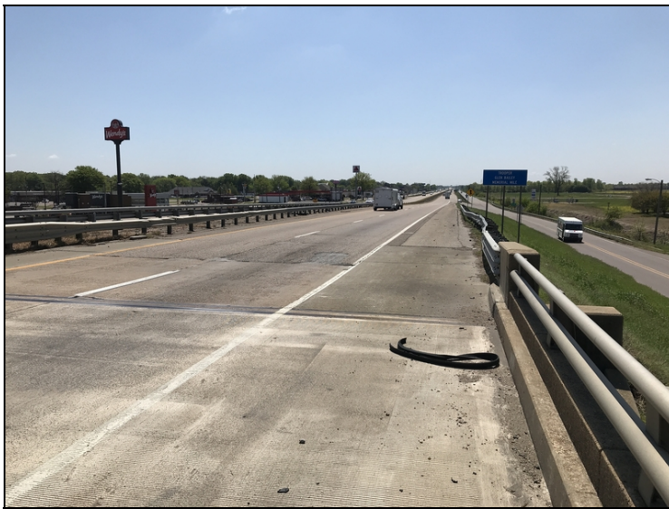
Abutment #1 both approach rails have collision damage.
