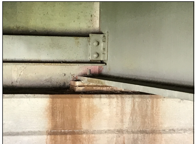
Typical abutment bearing nut missing.
