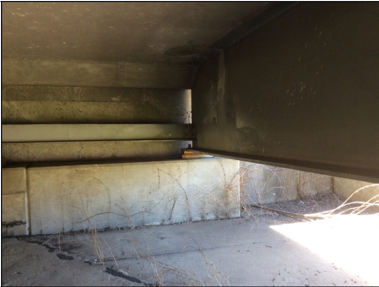
Typical bearing nut missing.
