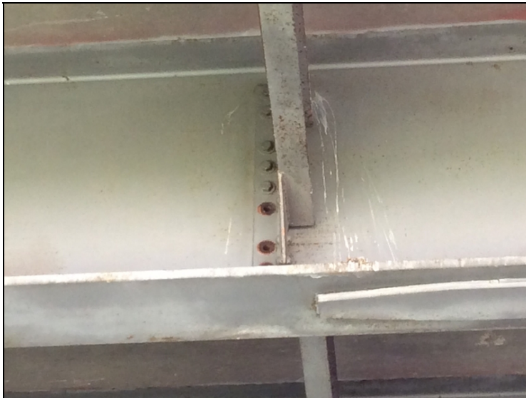
Typical diaphragm bolts missing.
