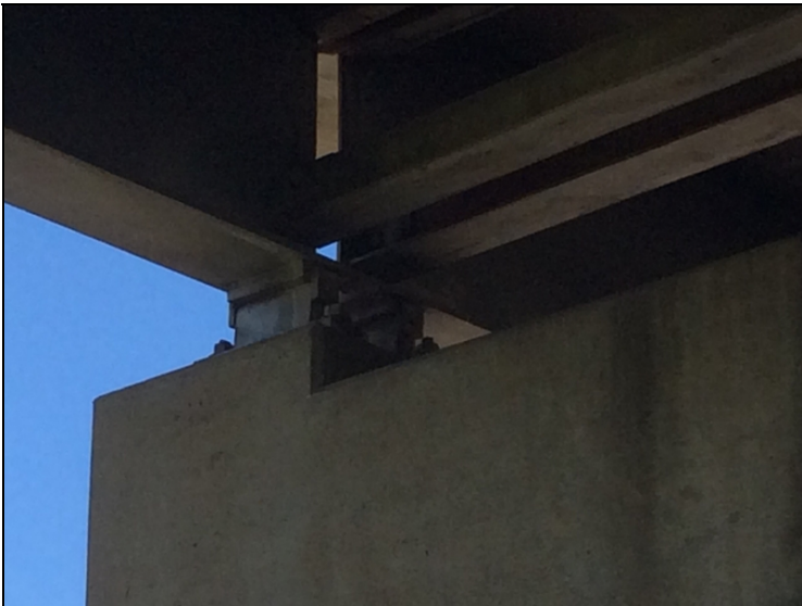
Typical girder to bearing bolt missing.
